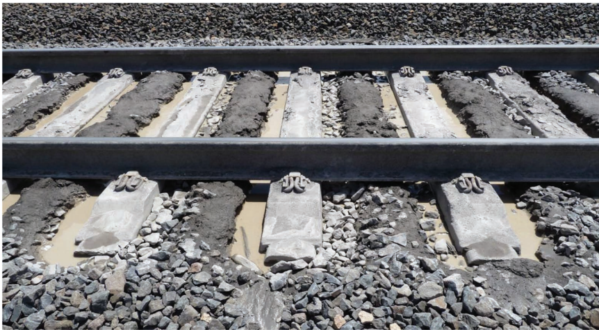
Figure 2.2 Section of track fouled ballast and poor drainage (courtesy of Australian Transport Safety Bureau, 2012)
